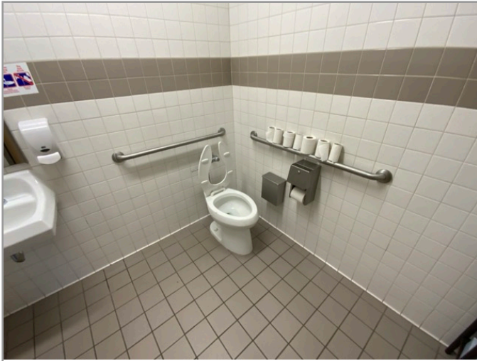
TOILET STALL OVERVIEW
