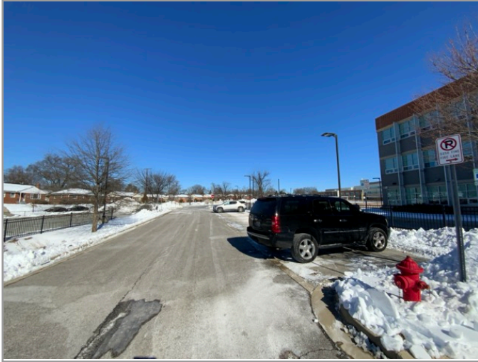
OVERVIEW OF ACCESSIBLE PARKING AREA
